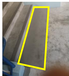
Figure 3 – Anti-slip paint at staircase landing
