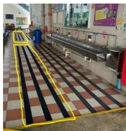
Figure 2 – Additional Anti-Slips at the canteen
